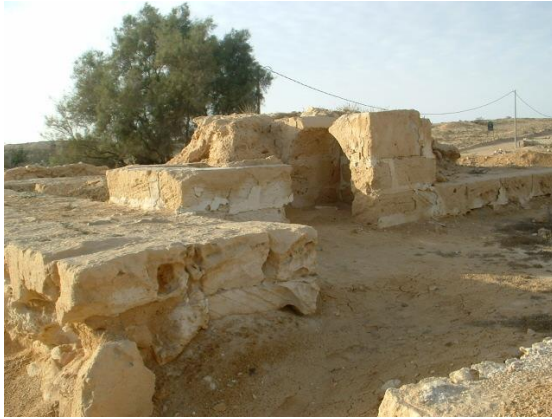
Fig.4 The tower's ground floor A square bolt-hole in the door-jamb is remarkable
